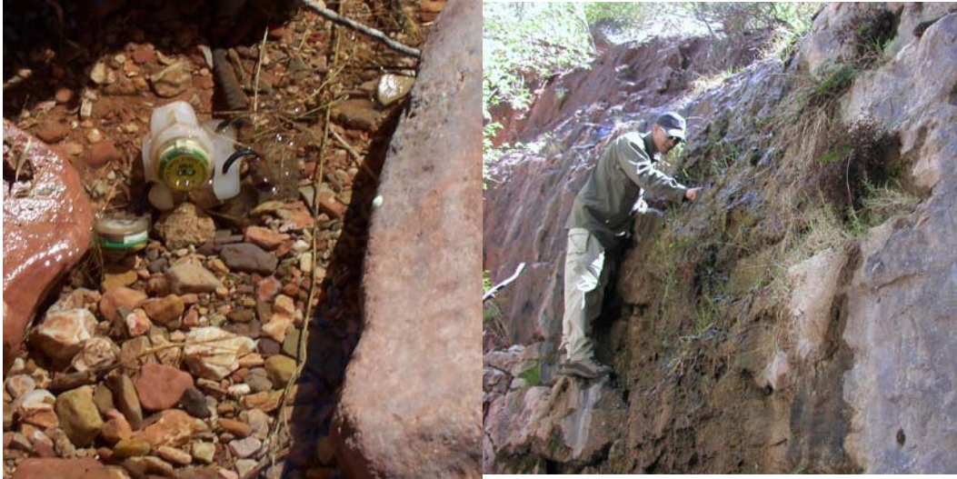
Figure 7. Photographs showing typical electrical resistance sensor installations; (A) Alluvial channel; (B) Rock wall.
