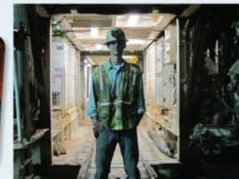
Alumnus Erik Hornaday in the Lake Mead Intake Tunnel. Photo by Charlie Schlinger.
