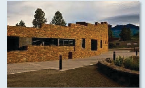
Museum of Northern Arizona Collections Building
