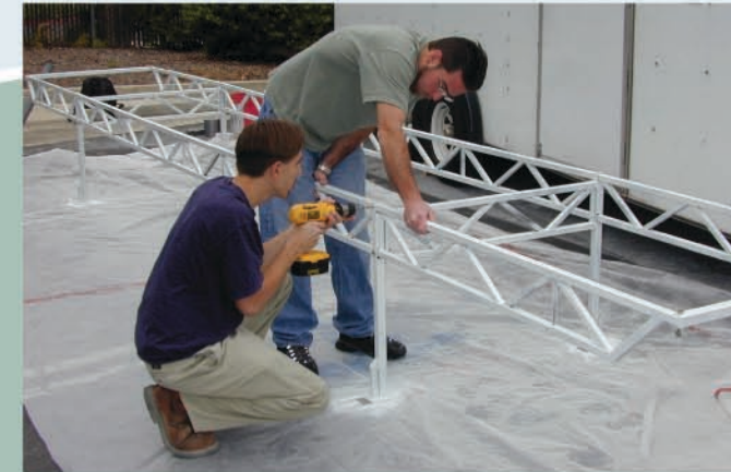
Assembling a bridge
