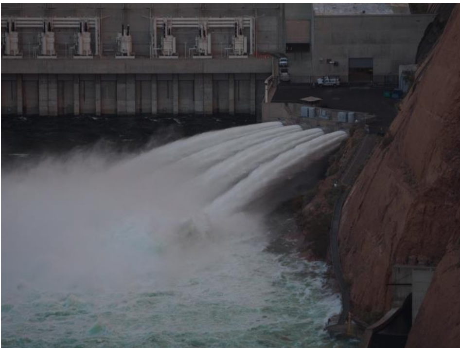
Open spillways at Glen Canyon Dam during a high flow event (artificial flood)
