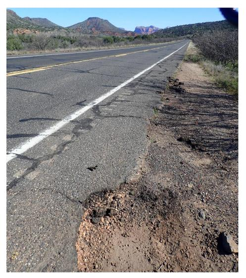
This image shows a section of narrow, eroded road shoulder along highway 179. The picture was taken looking northbound roughly 3 miles south of the Village of Oak Creek. Directly to the right of the white line in the foreground a rumble strip limiting the width of the shoulder for bike tires can be seen.
