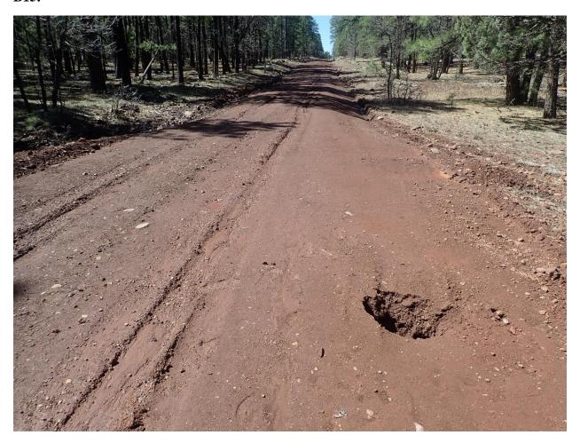
This picture shows a hole in the road where a metal corrugated culvert pipe for drainage caved in. The pipe runs perpendicularly under the road and appeared to collapse due to vehicles traveling on the road with the wet soft conditions.
