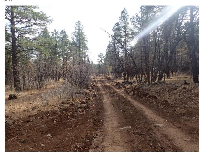
This photograph was taken by the field researcher looking south on Forest Road 132D. It shows a section of road that appeared to be hastily graded possibly during wildfire mitigation. Though it may not appear significant the rocks dislodged by the grading made this section painstakingly slower than the rest of the route.
