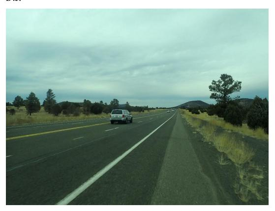
Wide shoulder along Route 64 where the speed limit is 65 mph and the road switches between 2, 3, and 4 lanes. The shoulder is this wide for roughly 70% of the distance between Spring Valley Road (forest road 141) and Interstate 40.
