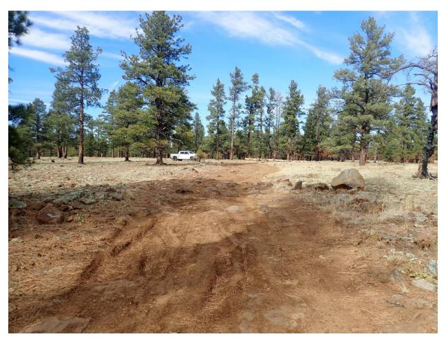
This photo illustrates the transition to the less maintained portion of Forest Road 132D once inside the Pinegrove Quiet Area. Particularly note the significant ruts and medium size rocks on the road surface.
