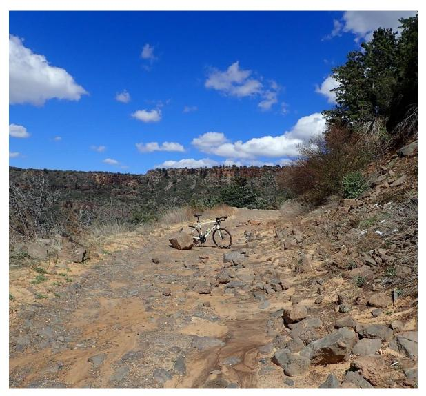
This image shows one of a few rockslides on Schnebly Hill road above the seasonal vehicle closure. The rock debris is seen on the right side of the road and the field researcher's bicycle is leaning against a large boulder that was likely part of the rockslide to provide scale.
