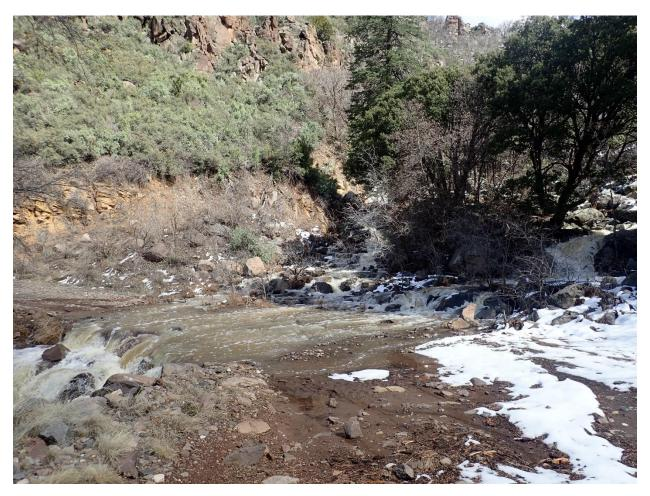
This picture shows Casner Canyon 1 on Schnebly Hill road taken on 3/21/2020. The water was flowing quickly and eroding the road. The water is crossing the road perpendicularly on a hairpin corner and is roughly 20-30 feet wide and up to 36" deep in places. The water depth looks minimal in the photo. The field researcher found this depth out the hard way when he attempted to cross the flow by bike.
